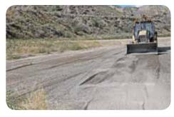
Gravelling the parking lot. A French drain was installed at the entrance to the lot to reduce surface runoff onto the lot.
