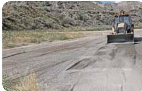
*Gravelling the parking lot. A French drain was installed at the entrance to the lot to reduce surface runoff onto the lot.*
